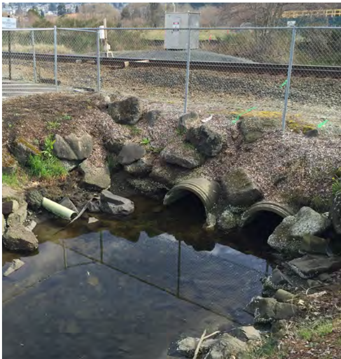
EXISTING WILLOW CREEK CULVERT
