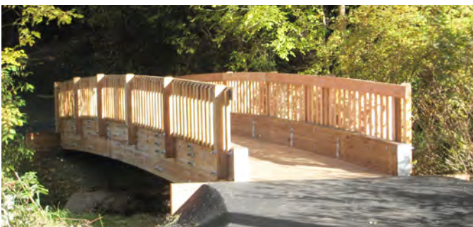
PEDESTRIAN BRIDGE EXAMPLE
